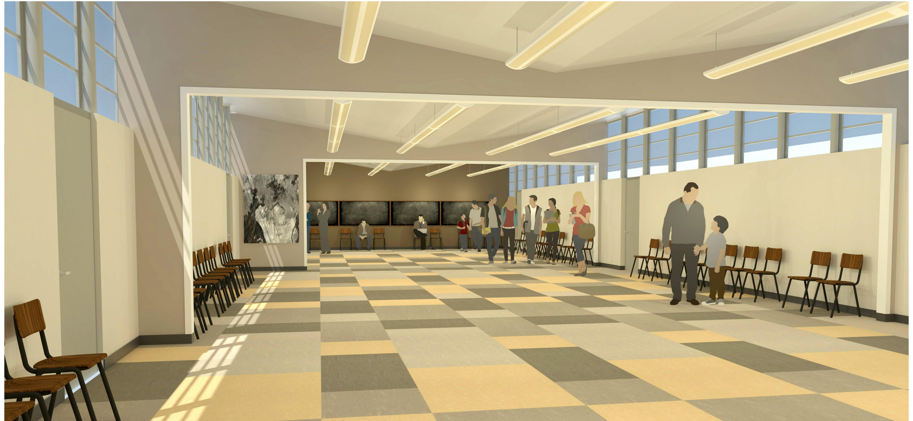
Armstrong suspended drywall system with Prudential 'Wave' light fixtures
