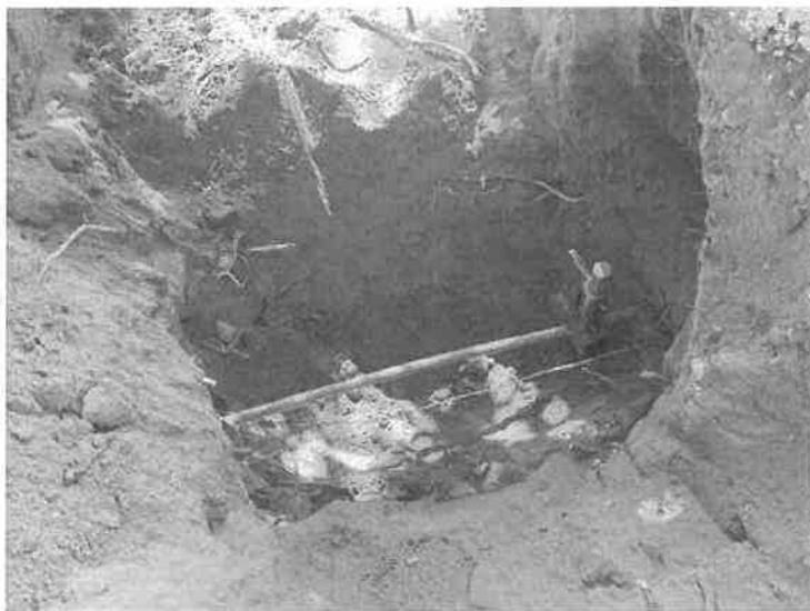
Photo 2 provided by Southern California Gas Company depicts the half-inch natural gas line. (Exh. 1.)
