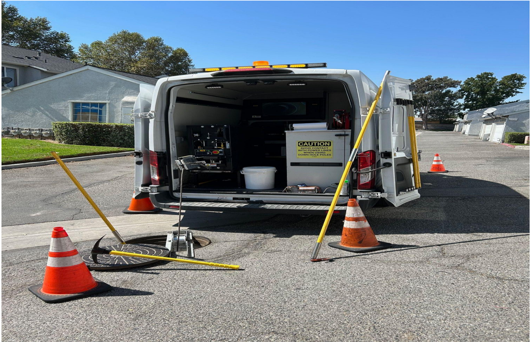
Camera Van inspecting sewer line
