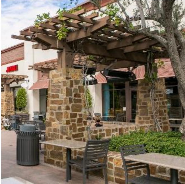
Example, Substantial and Durable Columns
