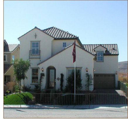
Recessed second floor
