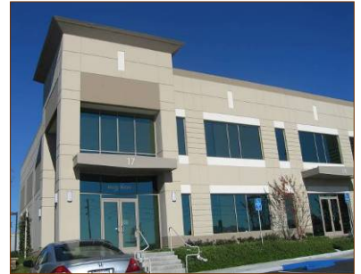
Typical painted finish articulated for pedestrian scale.
