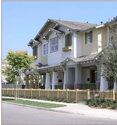
Exposed rafter tails
