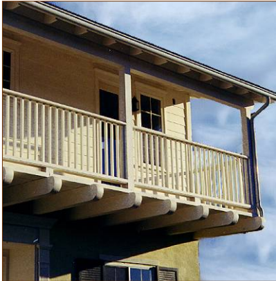
Cantilevered balcony with articulated floor joists
