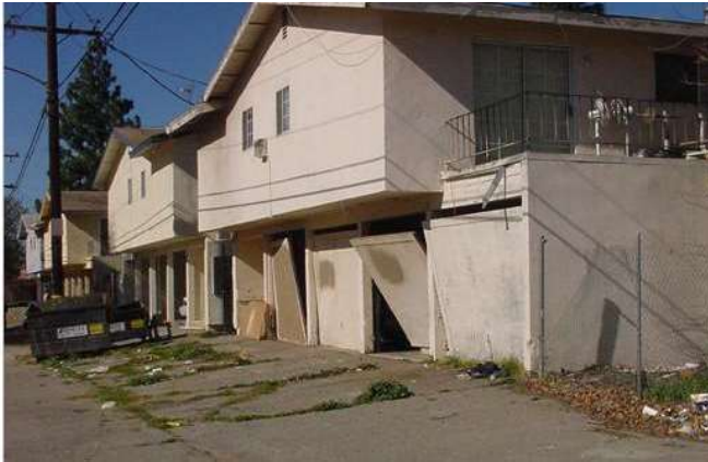
Prior to rehabilitation
