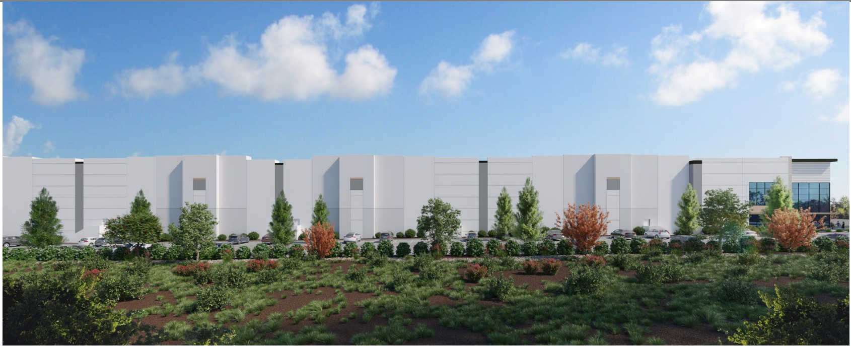
VIEW FROM EAST SIDE OF BUILDING FACING WEST
