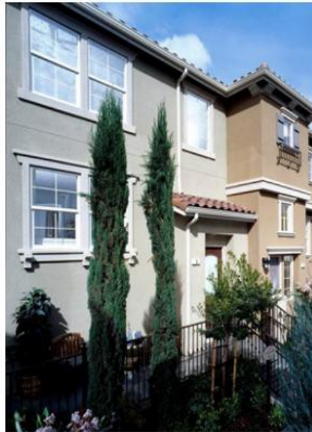
Example, Grouped Windows with Unifying Header and Sill
