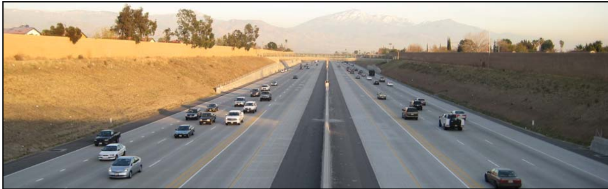
SR-210 freeway through Rialto
