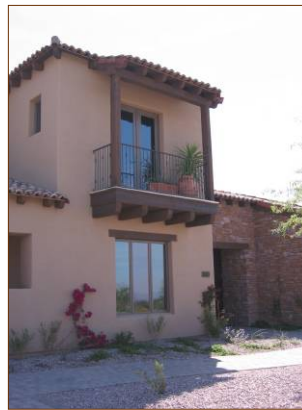
Balcony with decorative metal railings
