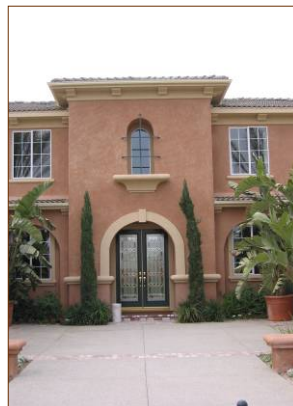
Dentils at eaves
