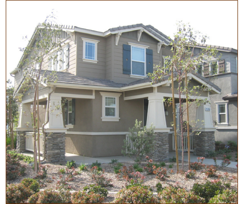
Battered columns with stone base
