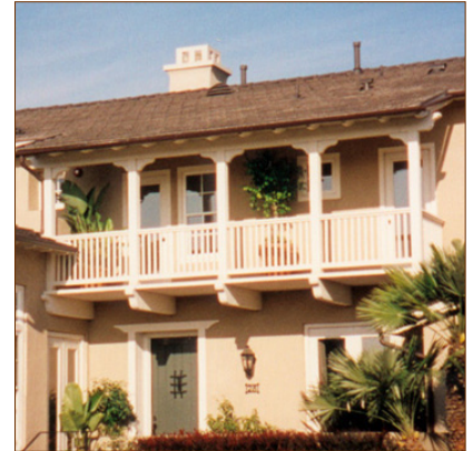
Exposed rafter tails
