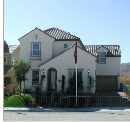
Recessed second floor
