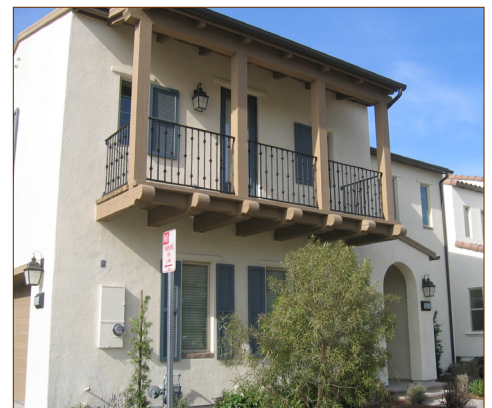
Wood corbels with decorative metal balcony railing
