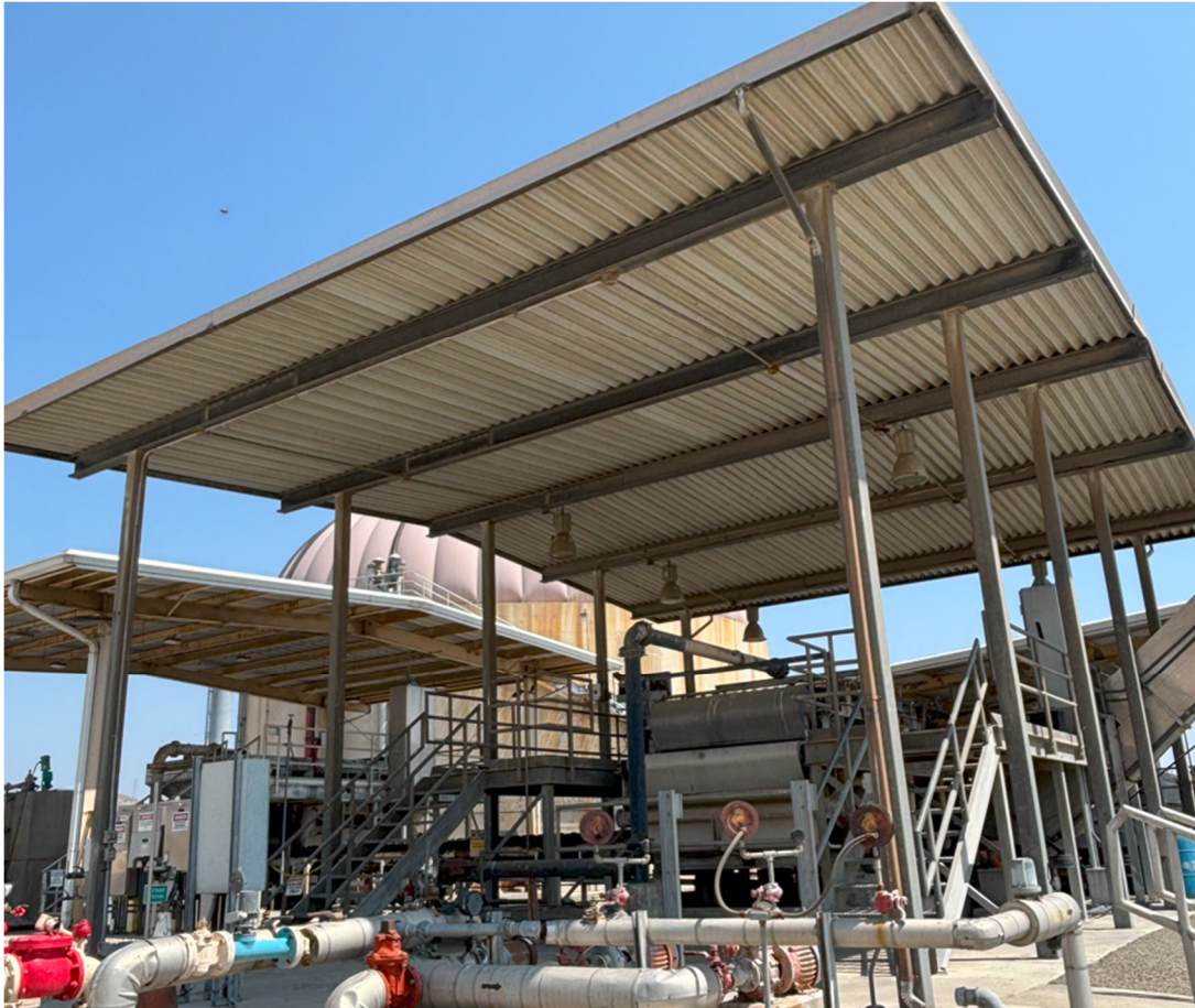
Figure 2 Overview of BFP 1 Facility (Facing Southeast)
