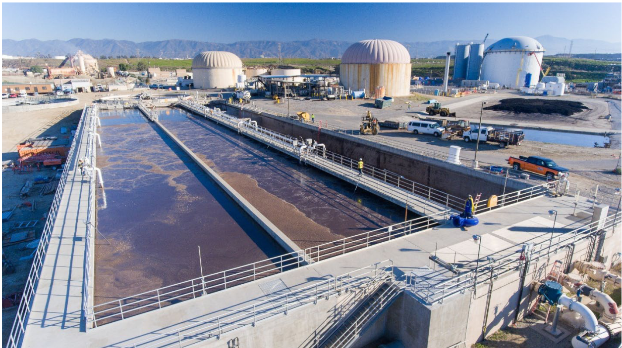
Existing biosolids processing facilities at the Rialto Wastewater Treatment Plant where upgrades will improve sludge thickening, digestion, and dewatering operations.
