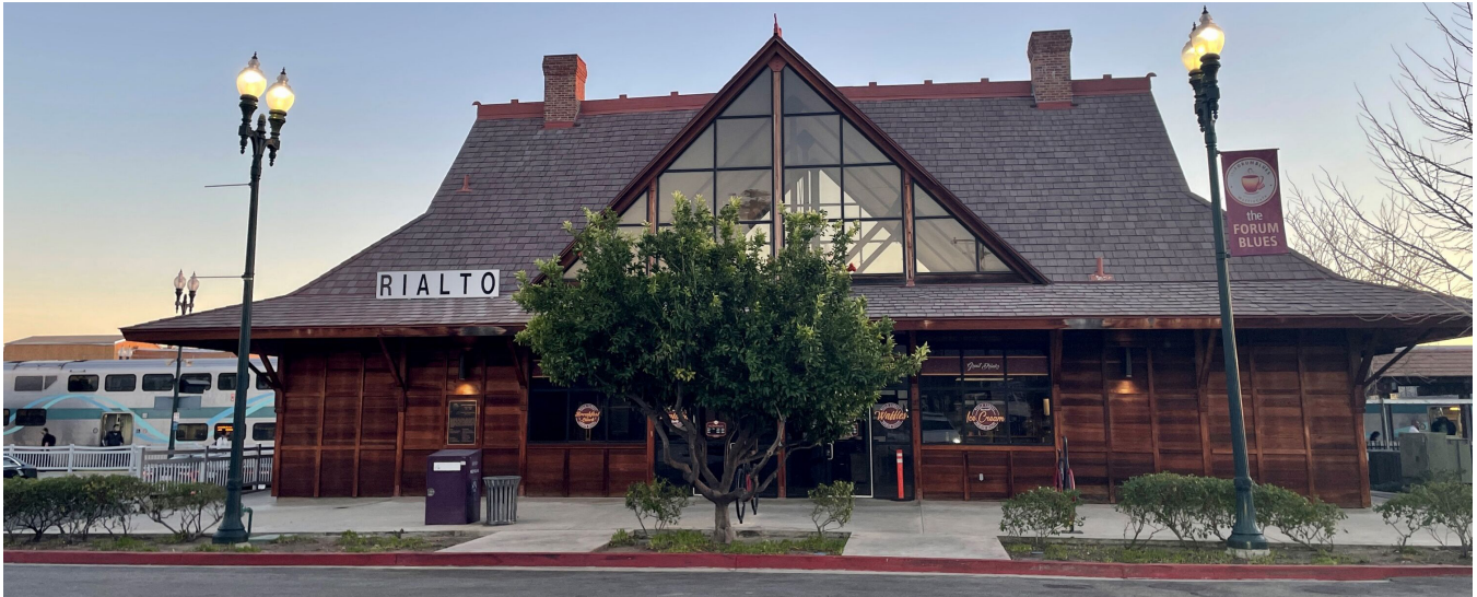
Quality architecture that draws on Rialto's history and culture can help create a focal point and sense of place.
