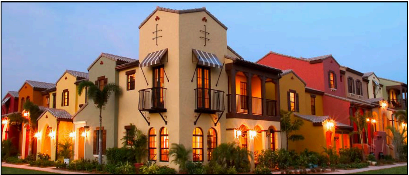
Below: A multi-unit building shares a similar architectural style with other units and includes private, ground-level entries that reinforce street frontages.
