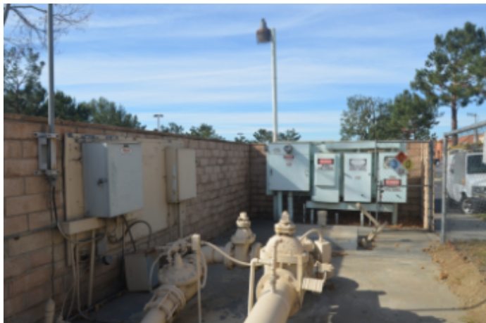
Figure 8 - Bypass 2 View of RTU to the Left and Control Panels Ahead
