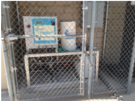
Figure 24 Existing Chlorination System
