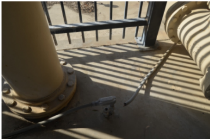
Figure 20 Wiring to instruments are disconnected and need rewiring.
