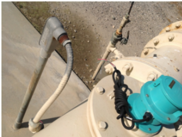
Figure 15 Existing Flow Meter to be Connected to PLC
