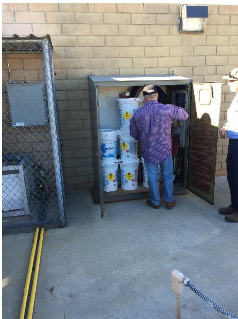
Chino PS #1 Chlorination Tablet Storage
