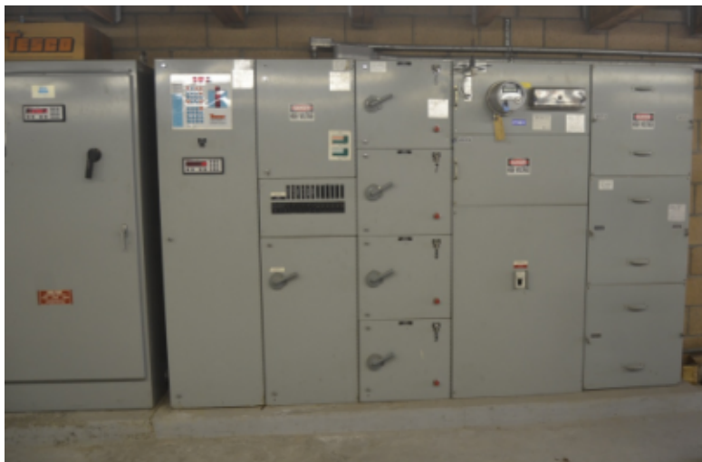
Figure 22 Motor Control Center for Boosters 6-10
