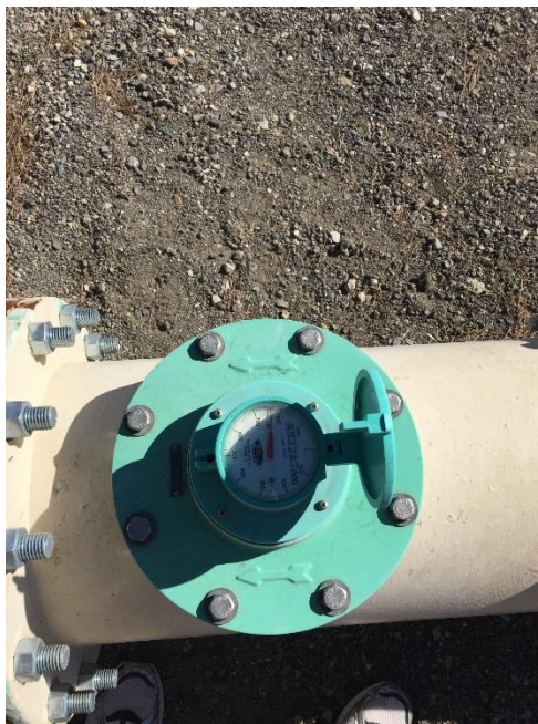
Booster 4 & 5 and Rialto Well #4 Flow Meter Details (1)
