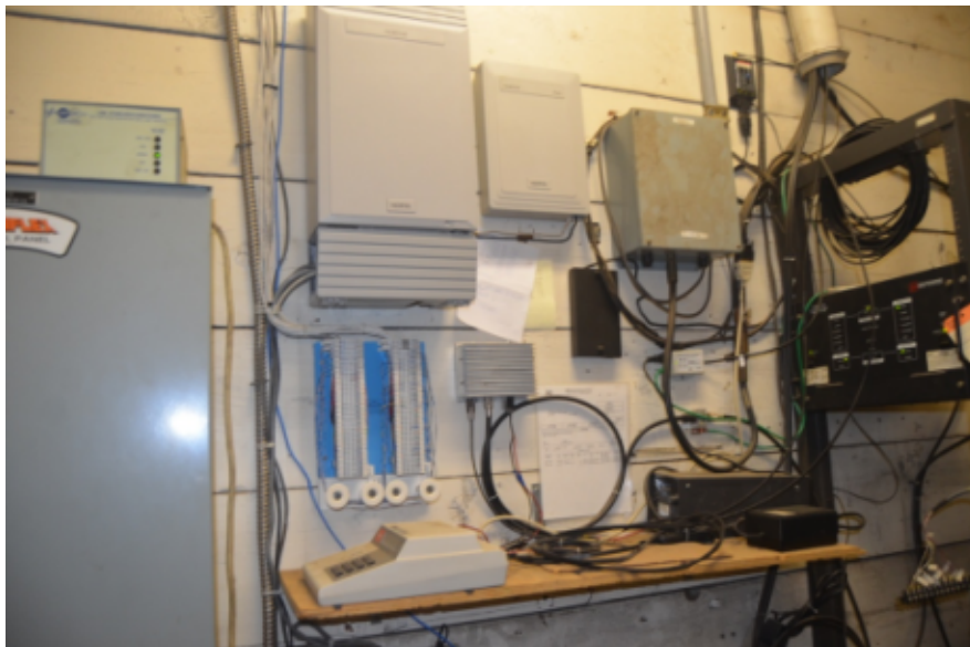
Figure 3 - SCADA Master Station Data Concentrator and Radio in new Server Room
