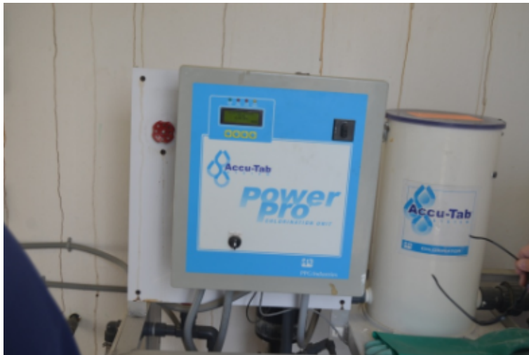
Figure 7 Chlorination Equipment to be Monitored.
