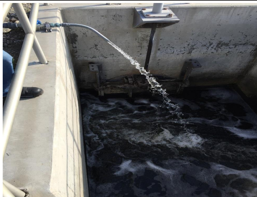
WWTP Chemical Dosing
