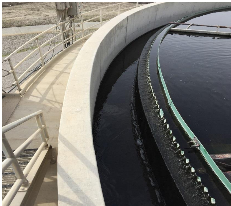
WWTP Plant #5 Secondary Settler
