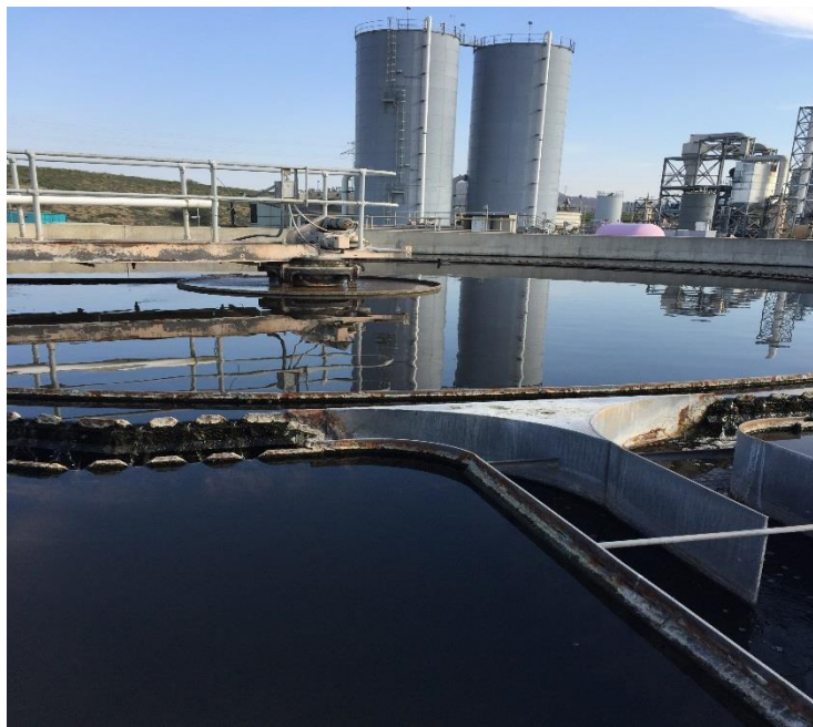
WWTP Plant #2 Primary Settler
