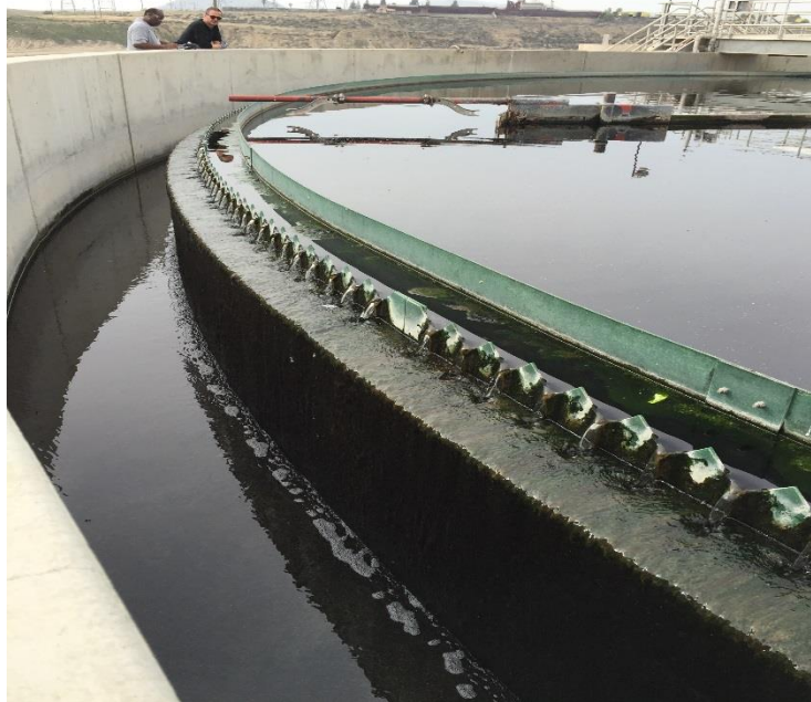
WWTP Plant #5 Secondary Settler (4)
