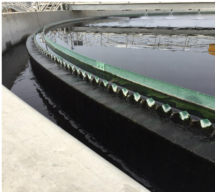
WWTP Plant #5 Secondary Settler (3)
