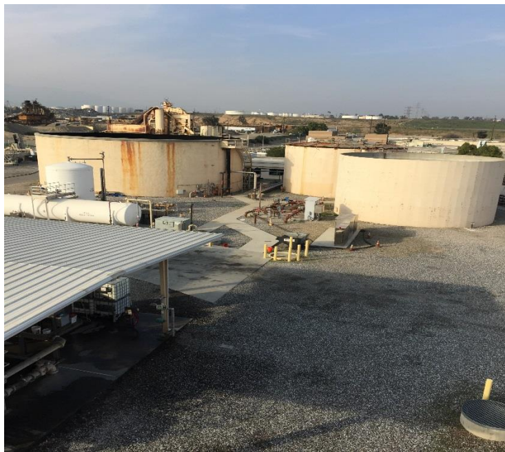
WWTP Digester #1 and Secondary Digesters
