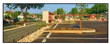
Parking Lot Improvements Projects (\$550K): Located in the City of Temple City, this project included new parking lot signage, asphalt resurfacing, construction of trellis, new lighting, electrical vehicle charging station infrastructure, landscaping, and drainage. Transtech provided design, construction management, and inspection services.
