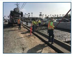
The project consists of cold milling existing AC pavement, tire rubber modified asphalt concrete overlay, remove and replace driveway approach, sidewalks, curb and gutter, alley intersection ADA compliant curb ramps, AC pavement, PCC pavement, (PCC bus pads, signing and striping, traffic signal modifications, and all other appurtenant work on Imperial Highway between Prarie Avenue and Van Ness Avenue.
